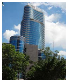
ZTE Central Office, Shenzhen
