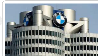
BMW Central Data Center, Munich
